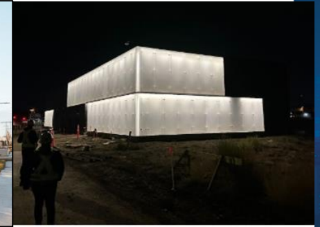
Night Shot of Blatchford Utility Complex
