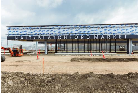
LRT construction continued
