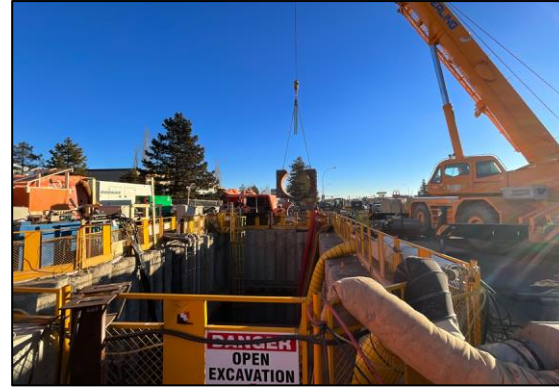
Launch Shaft Tunnel Operation
