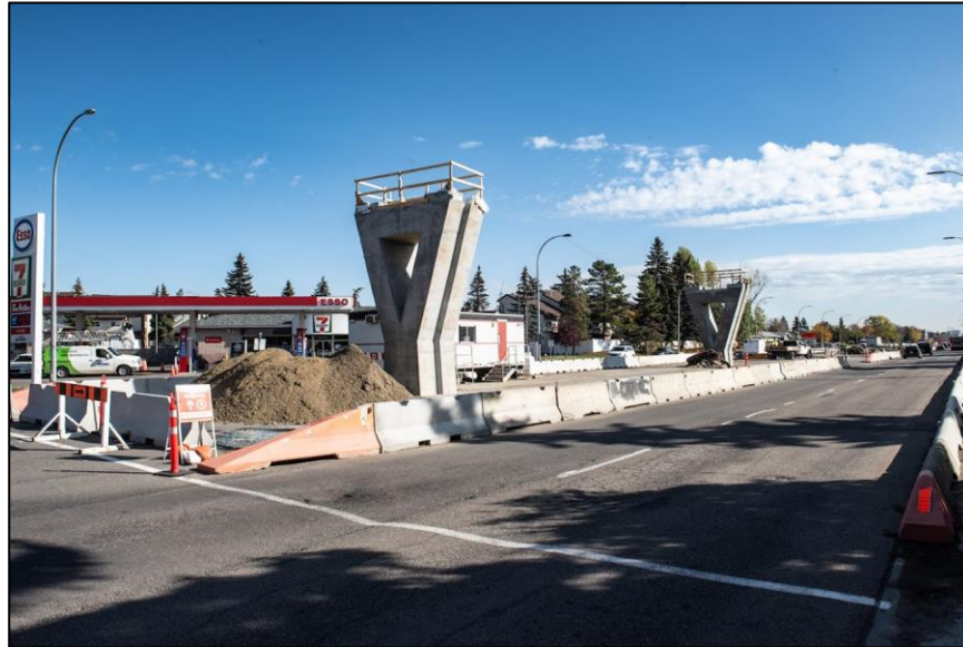
Elevated Guideway piers on 87 Ave
