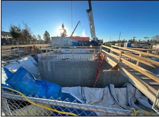
Lift Station Completion: June 2024
